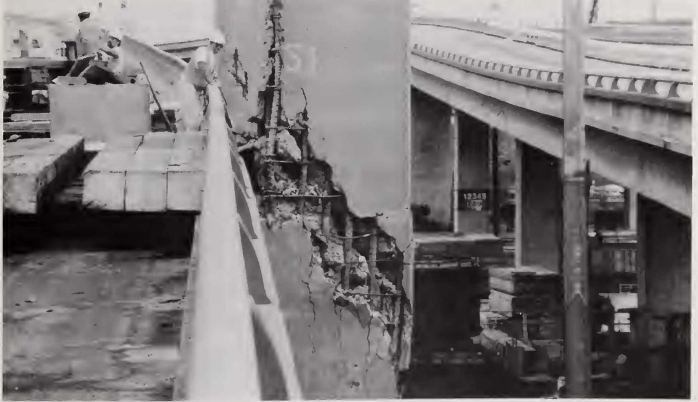
Figure 5.9.8 Diagonal cracking of the east-side column of Bent 51 (south face).
