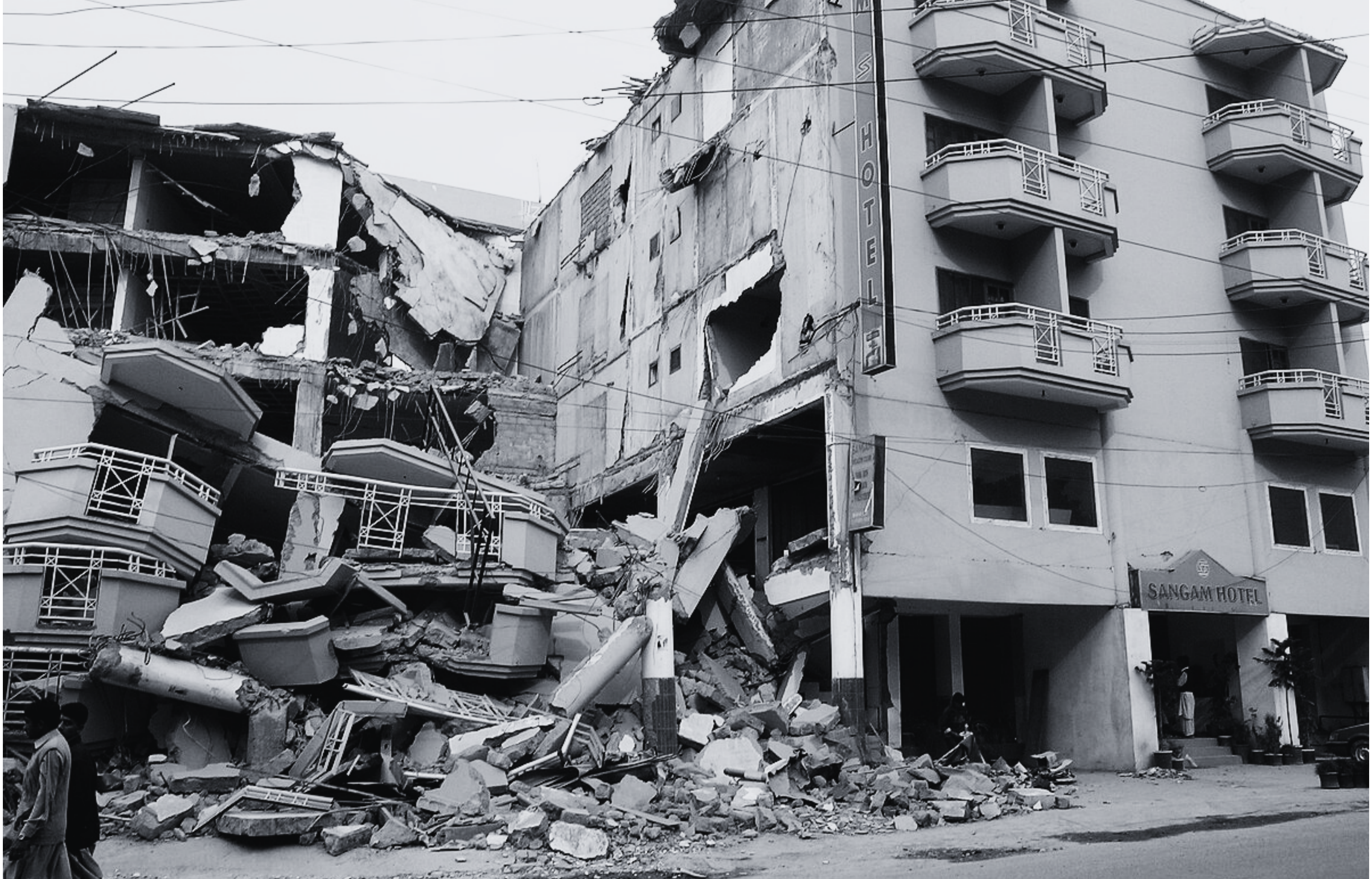
Destroyed building in Muzaffarabad after the earthquake, 2005.
